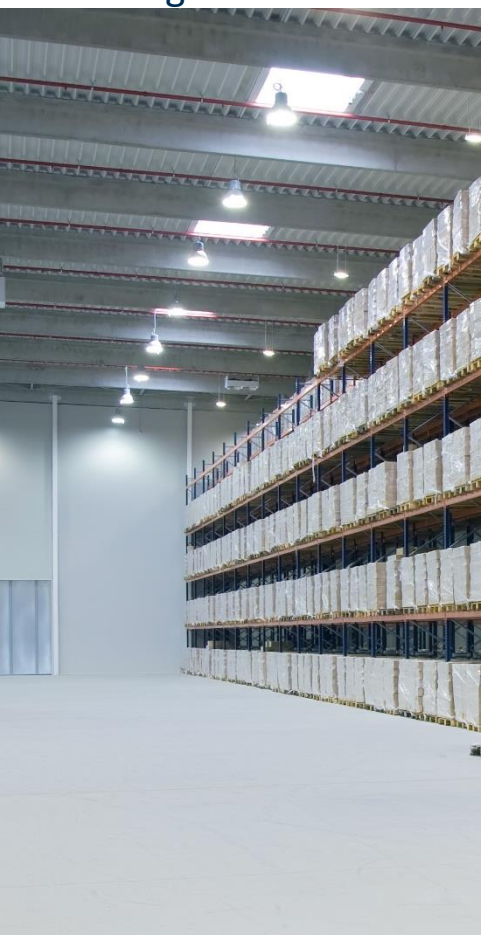
Warehouse Logistics hall
